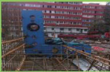
Rectangular(L) load cell
