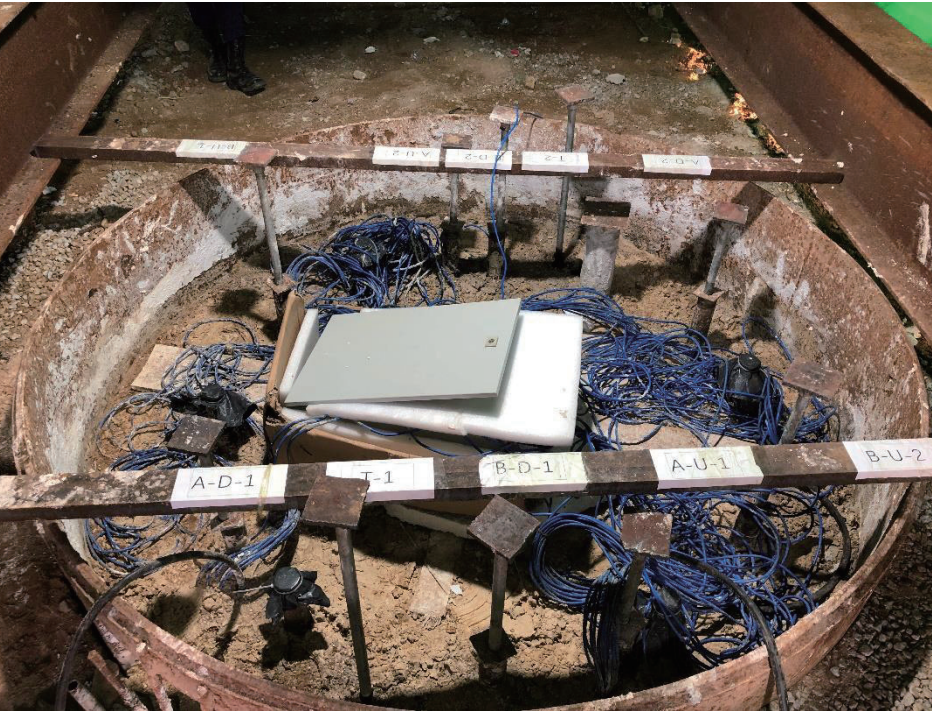
c) Marking at the pile head
