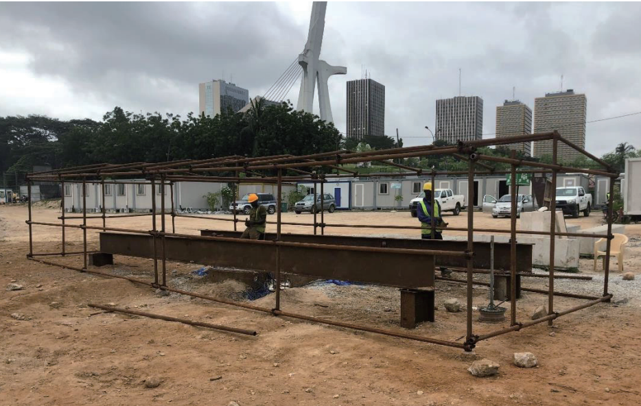
a) Erection of reference beams
