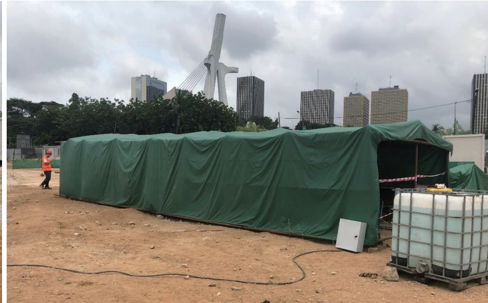
b) Erection of test shed
