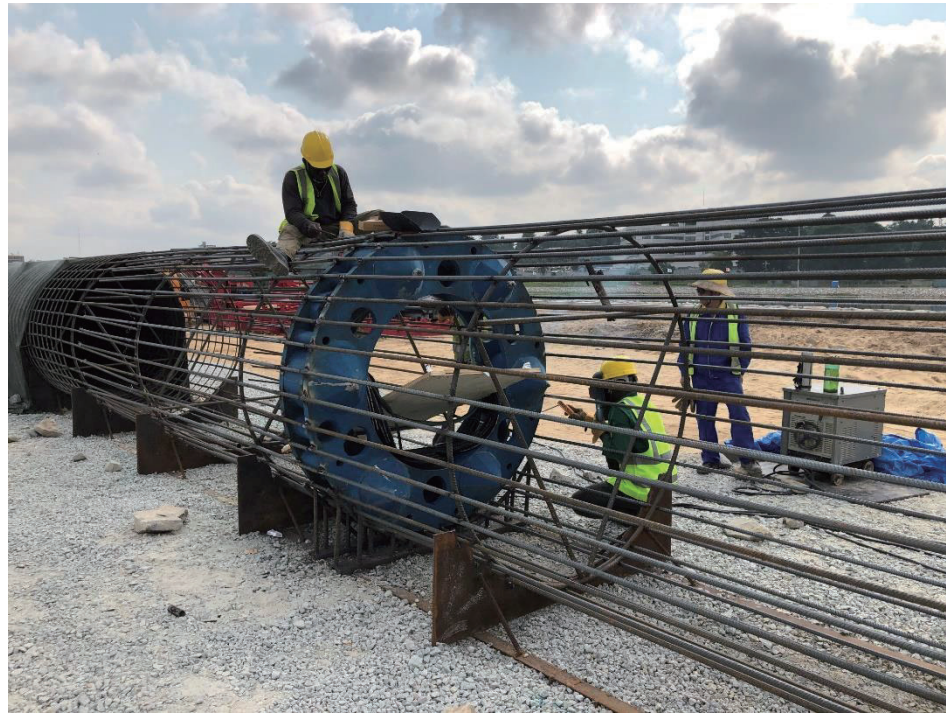
b) Welding with steel cage
